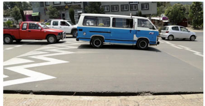
Speed management improvements included the installation of rumble strips (left) and speed humps (right). Photo source: Addis Ababa City Administration Traffic Management Agency.
